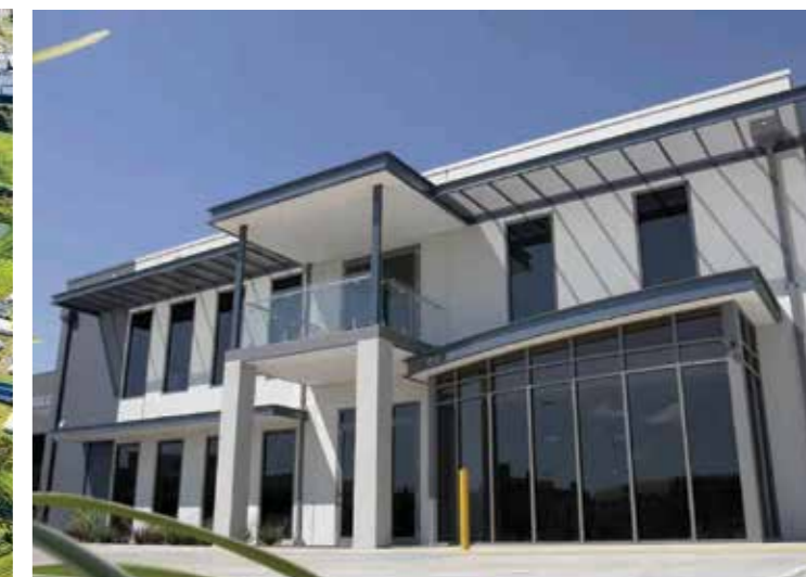
Forrestdale WA Facility
