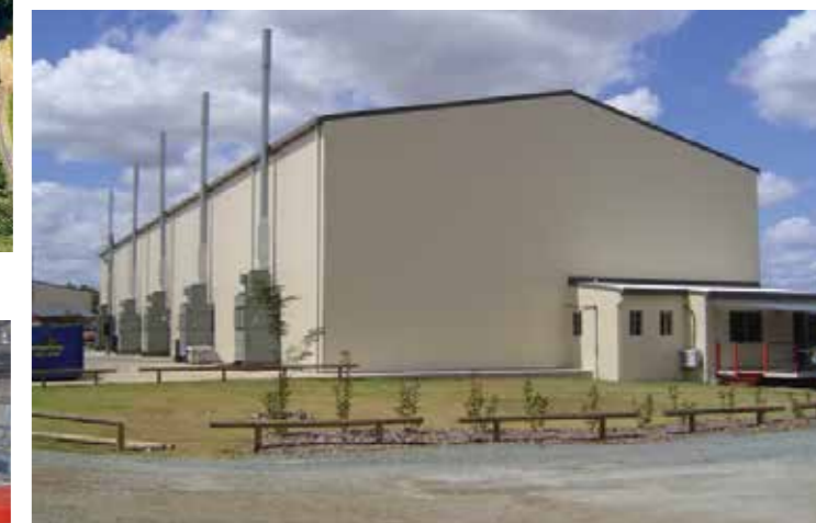
South Carolina USA Facility
