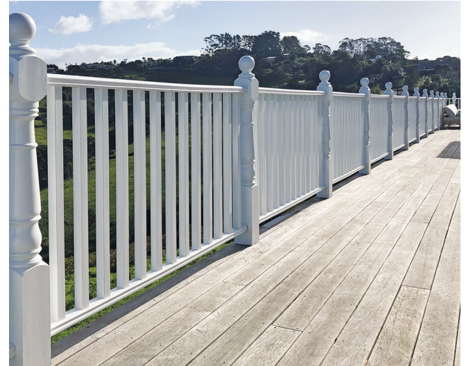
Villa 3: Villa Verandah with turned Balusters, Newell Posts, Handrail, Bottom Rail and Fillet:
