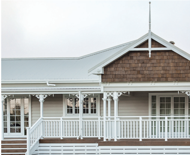
Villa 2: Villa Verandah with Collar Mould, Fretwork Brackets, Finial, Post Caps and Teardrops:
