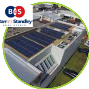
Barr & Standley 20kW System
