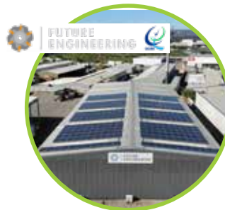
Future Engineering 100kW System
