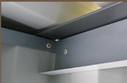
Folded heavy gauge channel, riveted for strength and durability.
