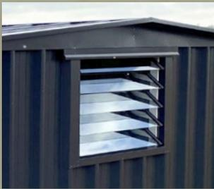
**Louvre window** allows natural light and airflow.
