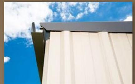
All our sheds have folded steel gutters to control water flow.
